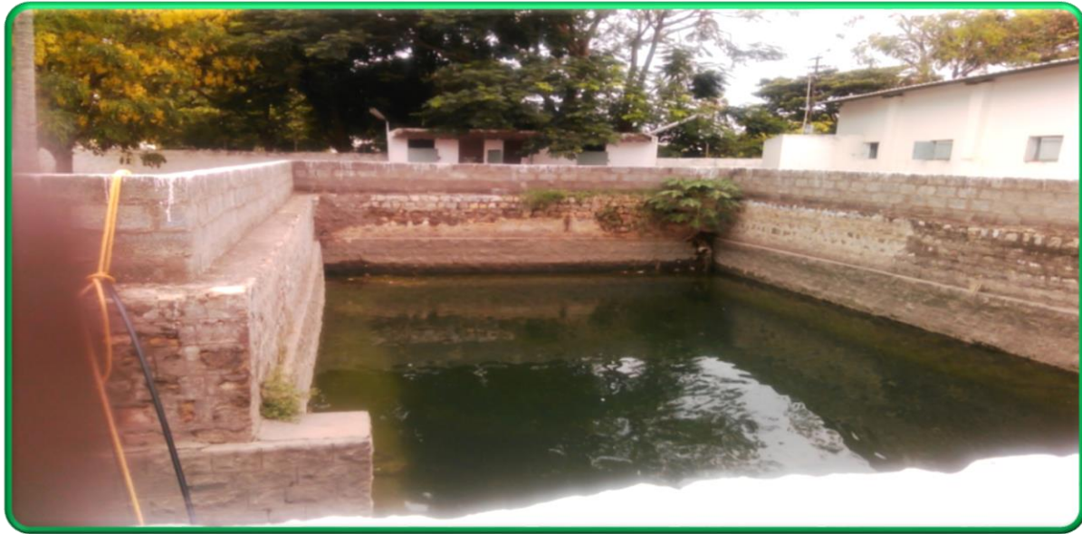
Huge Well with rain water harvesting facility:
